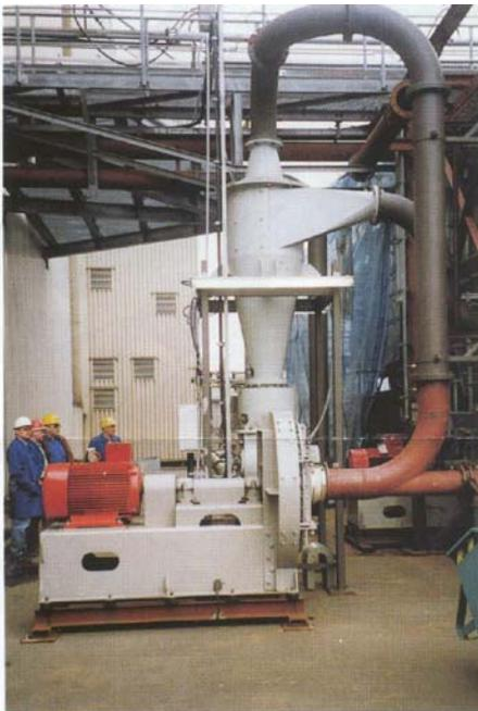
Fig. 3: Cyclone, fan and piping
